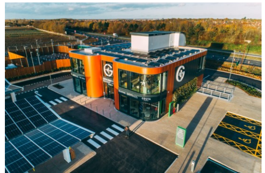
Figure 38: GRIDVOLT charging hub
