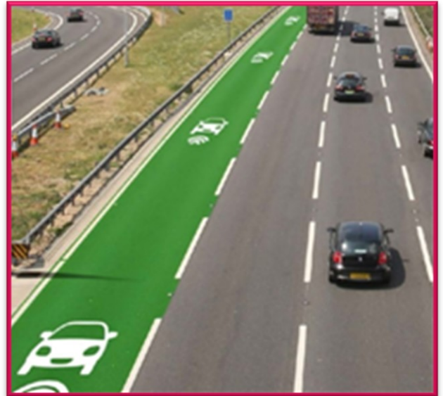
Figure 39: Wireless in road charging
